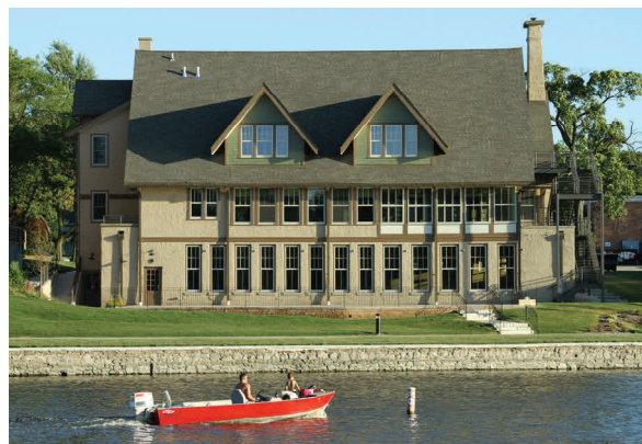
Restoration and renovation of the Fort Atkinson Club
